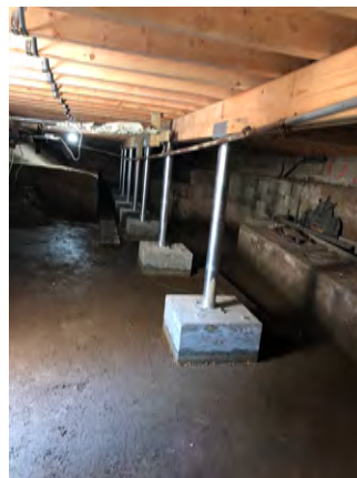
New galvanized columns
