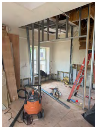
New closet rebuild
