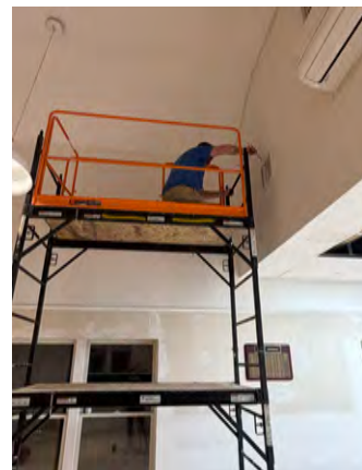
Volunteer crew painting interior
