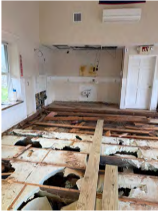
Ripping up old flooring
