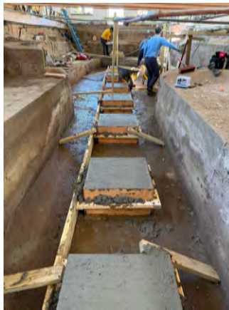
New forms being placed with rebar to support new columns
