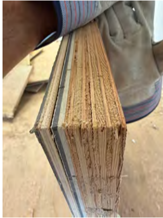
Ripping up old flooring
